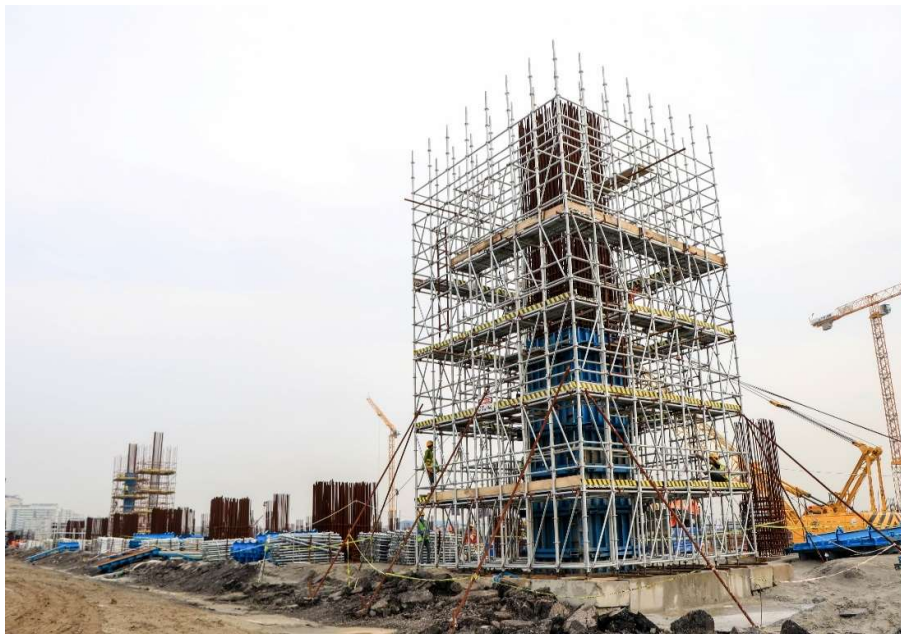
Figure 1.4: Scaffolding at construction site
