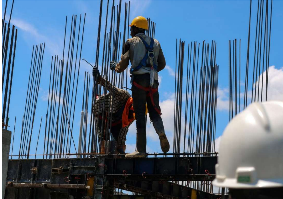
Figure 1.9: Working at height with safety harness
