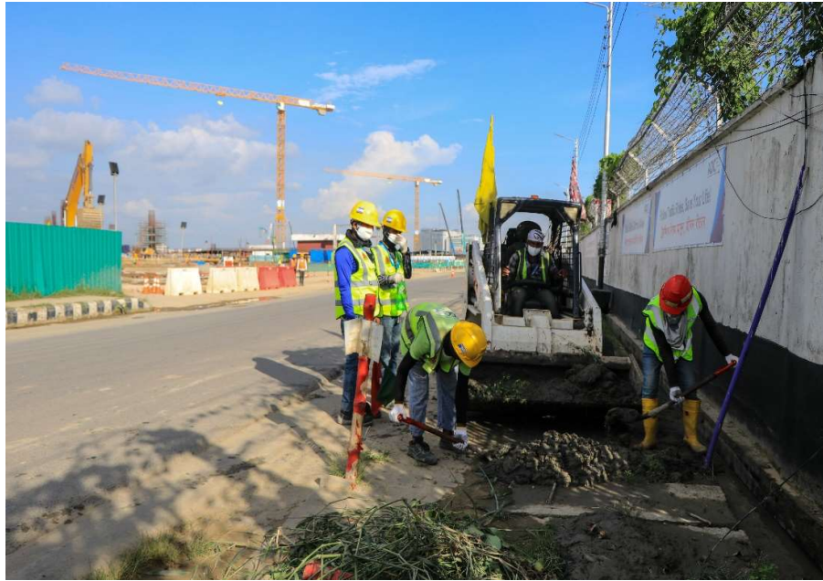
Figure 3.5: Removing waste from site
