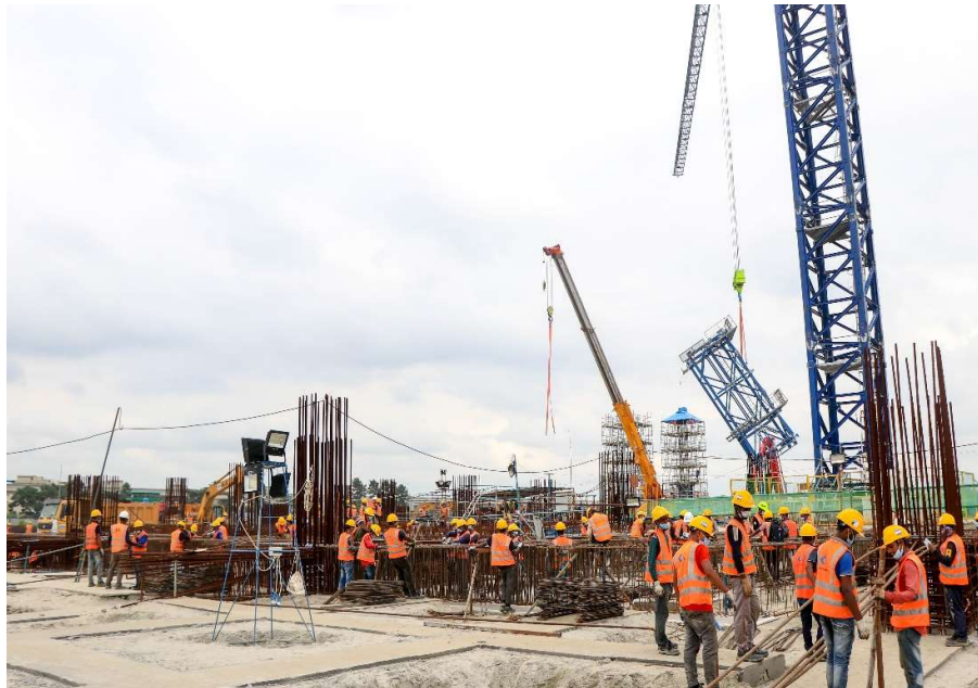
Figure 3.8: Worker working with proper safety
