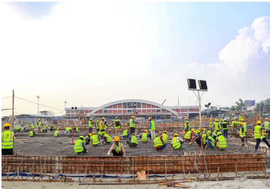
Figure 3.4: Worker working with proper PPE
