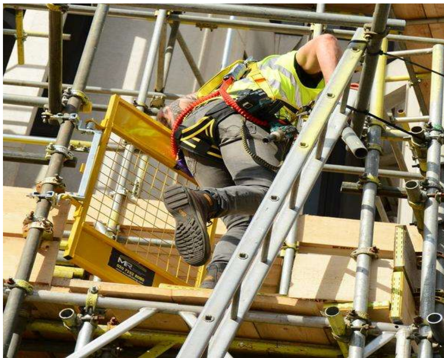
Figure 1.5: Correct use of ladder and safety harness
