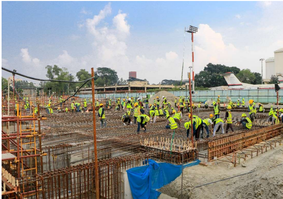
Figure 1.10: Worker Working with proper safety
