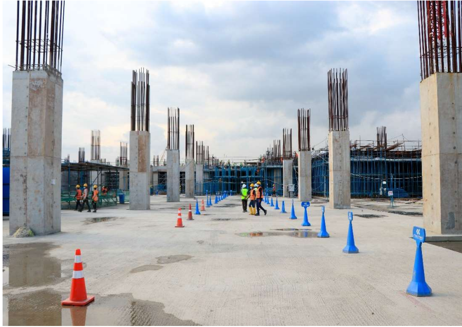
Figure 3.7: Proper Housekeeping at construction site
