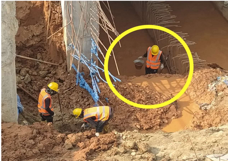
Figure 3.29: Without rubber gloves worker working at soft soil area
