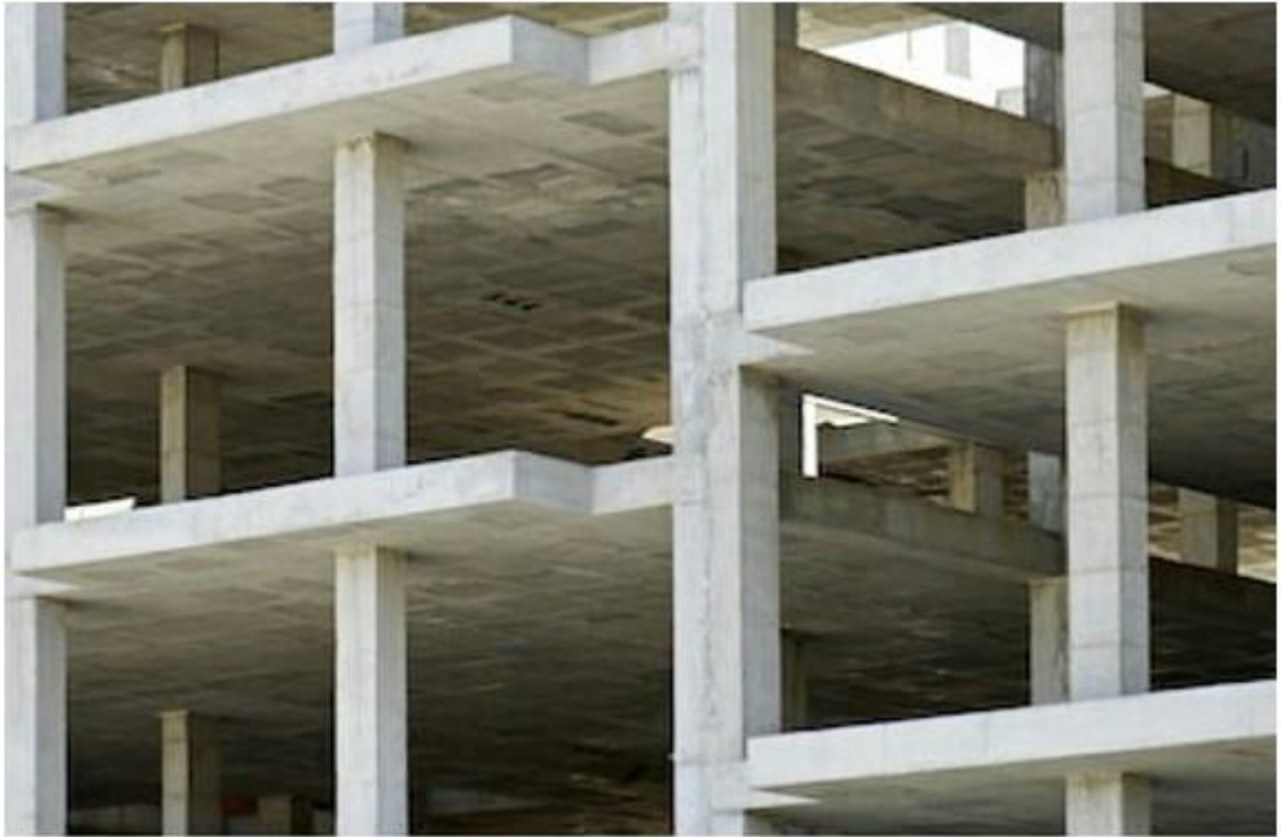
Figure 1.3 Flat slab floor system
