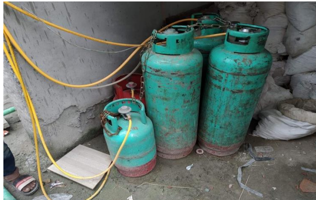
Figure 4: The gas cylinder in the ground floor
