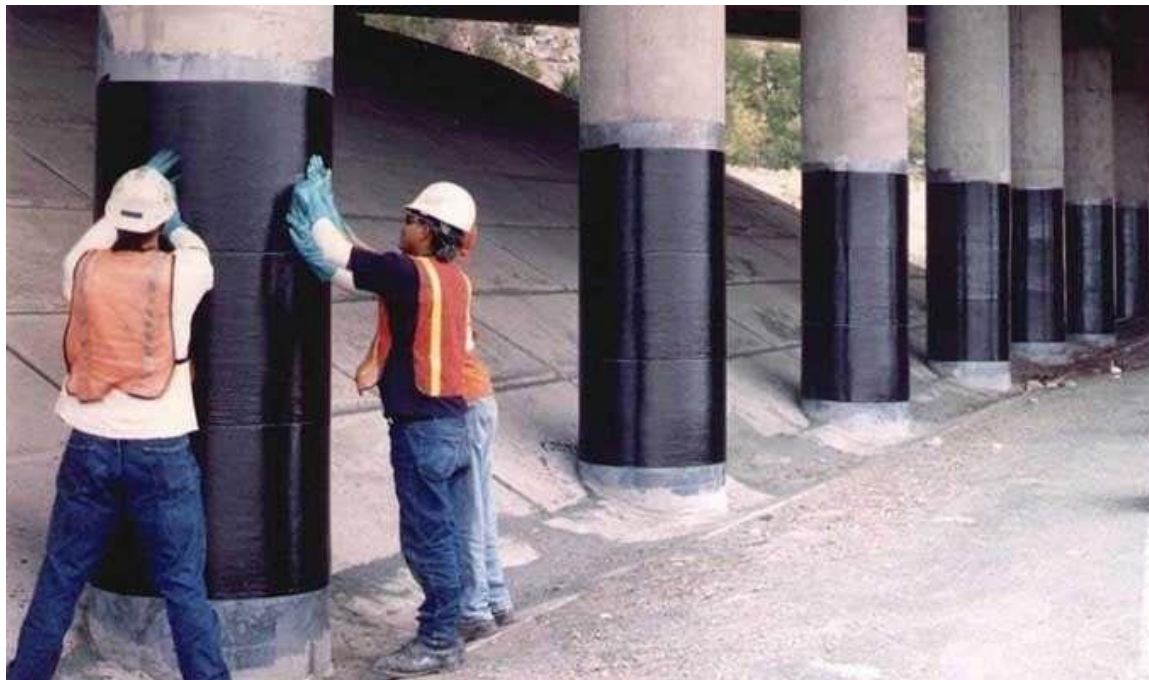
Figure 2.2: Fiber Reinforced Polymer (FRP) Wrapping
