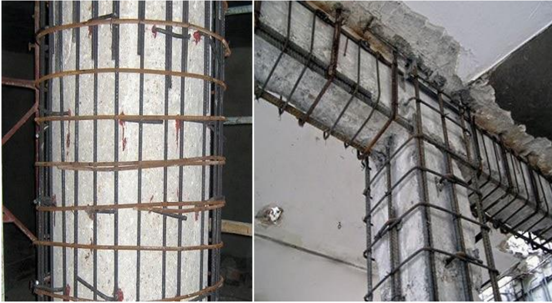
Figure 2.1: Concrete Jacketing
