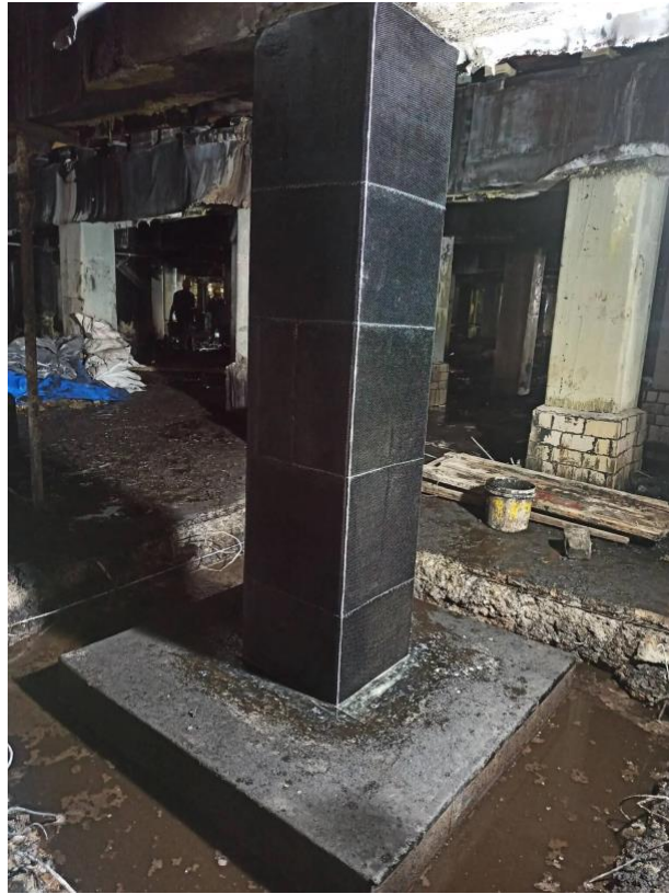
Figure 4-6. CFRP Retrofitting.
