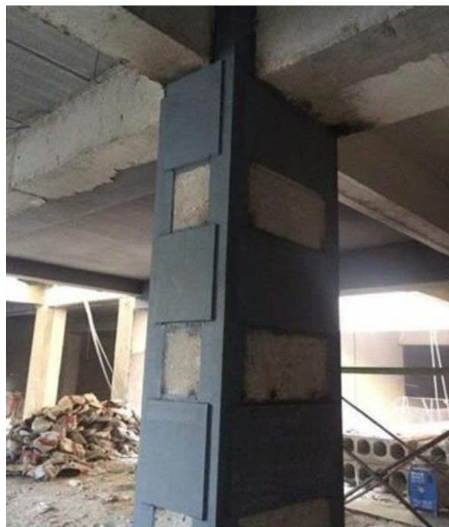
Figure 4-5 Retrofitting process of Steel plate.
