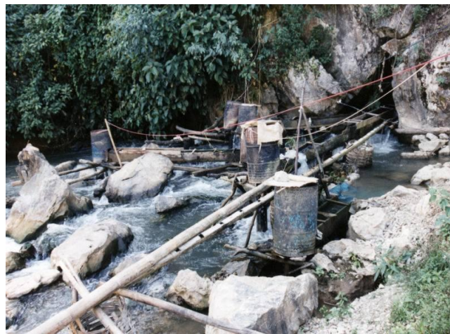
Fig. 2.2: A micro-hydro facility in Vietnam [vef]
