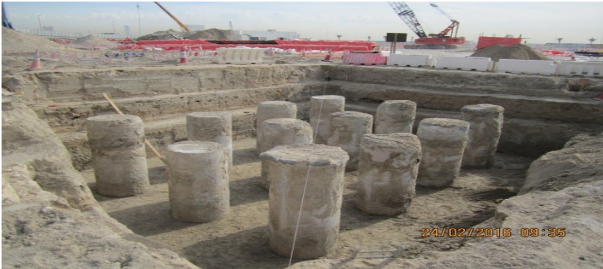
Fig.: 3.13. Excavation around piles
