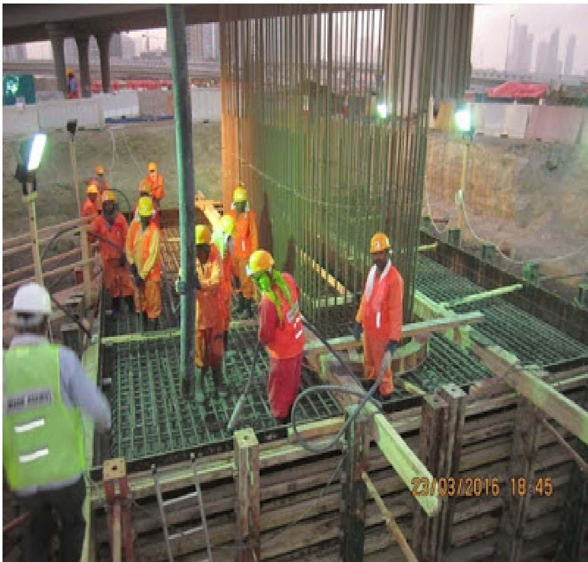
Fig.: 3.19. Concreting of the pile cap
