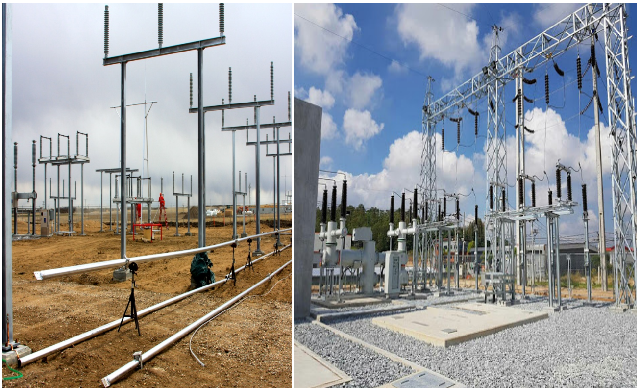
Fig.: 3.23. Assemble the steel structures
