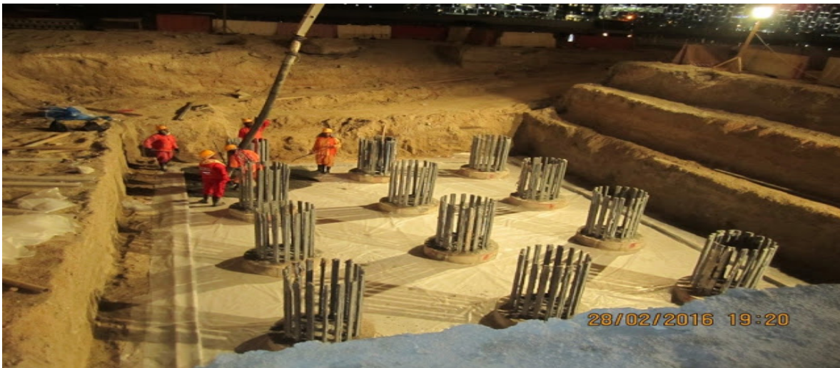
Fig.: 3.15. Preparation for lean concrete casting
