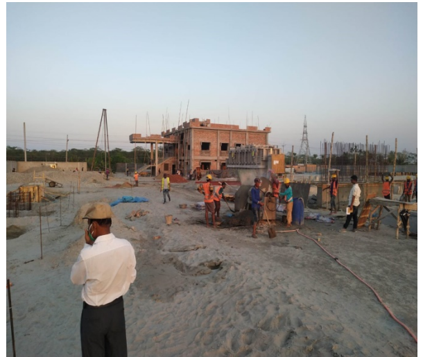
Fig: 4.7. Concrete mixing for casting
