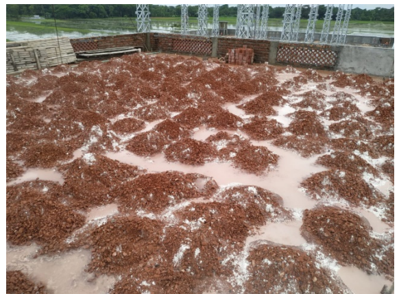
Fig:4.11 Lime terracing work on CRB slab
