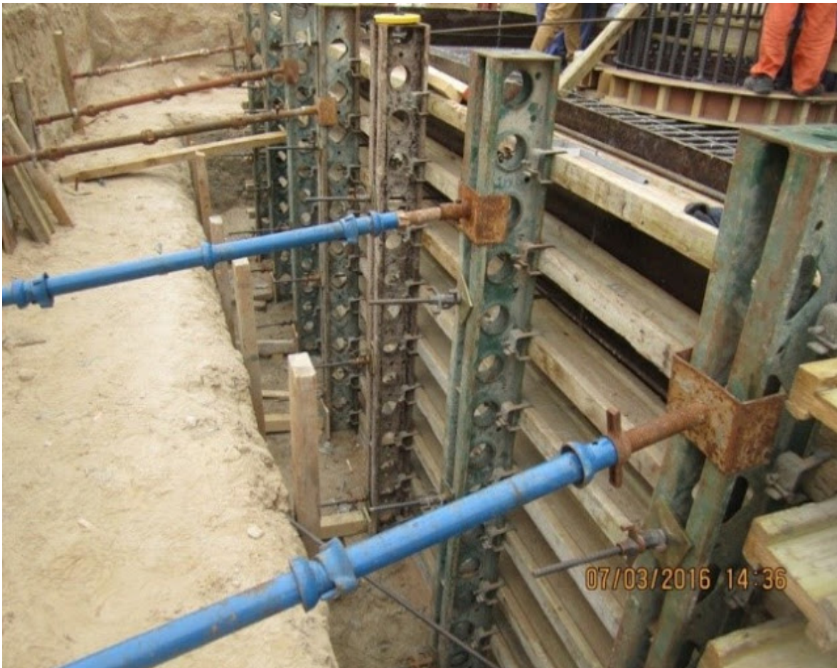
Fig.: 3.18. Formwork installation for pile cap
