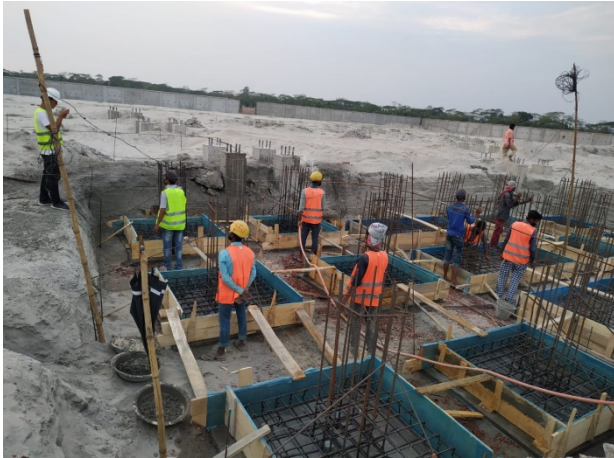
Fig: 4.2. Equipment base casting (LA, CT, CB)
