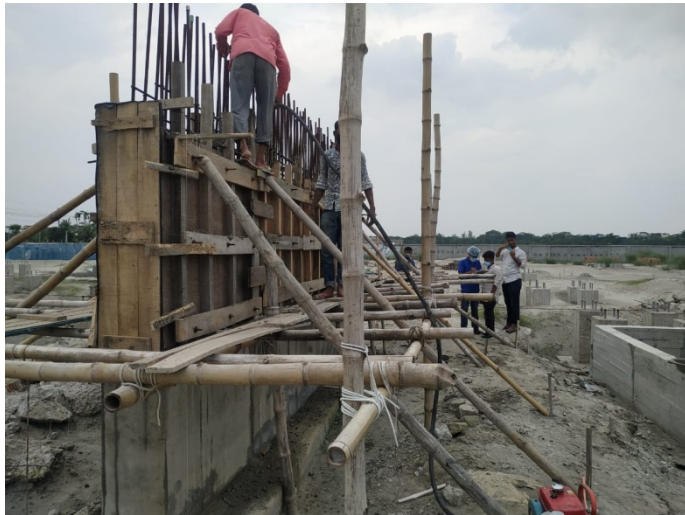
Fig: 4.6. Blast wall formwork setting & casting
