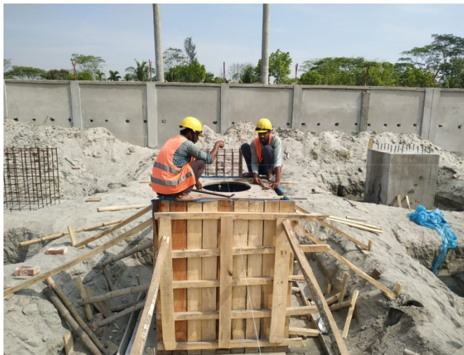
Fig: 4.4. Anchor bolt setting in short column
