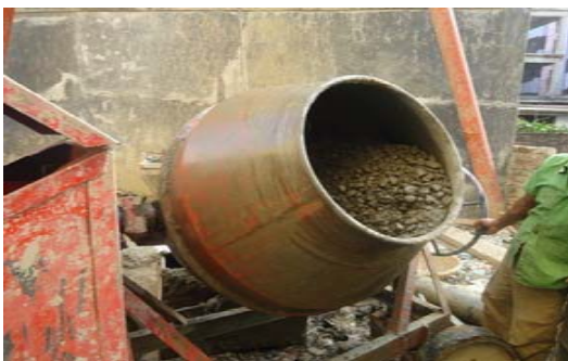
Fig: 3.7. Concrete mixing
