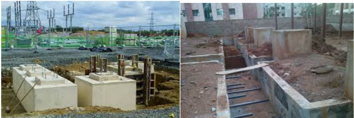
Fig.: 3.22. Backfill the foundations in substation yard
