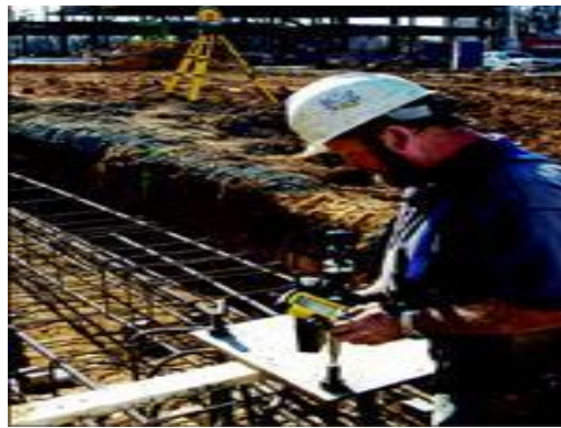
Fig.: 3.20. Layout for anchor bolts setting
