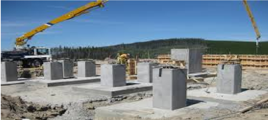
Fig.: 3.22. Backfill the foundations in substation yard
