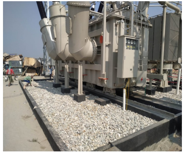
Fig: 4.15. Gravel laying on transformer pad
