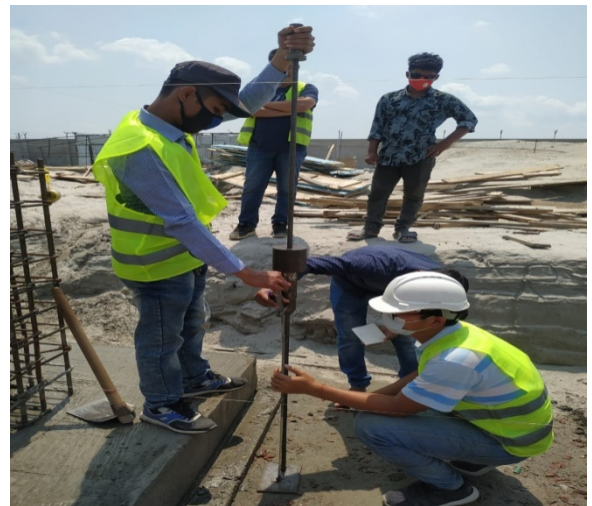
Fig: 4.5. Sand Compaction test
