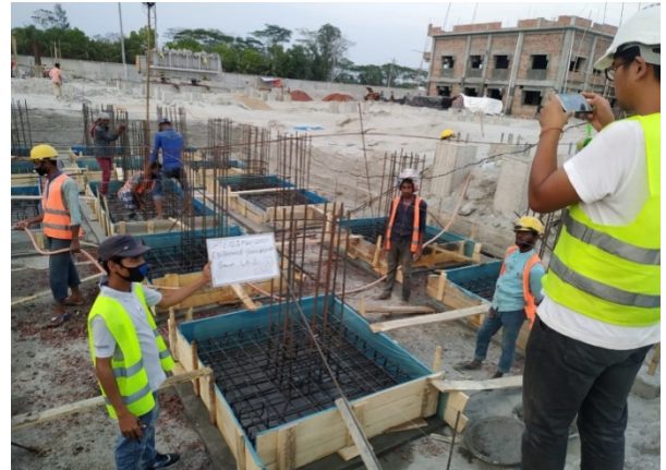
Fig: 4.3. Equipment base casting (LA, CT, CB)
