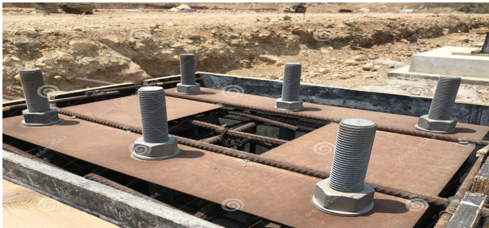
Fig.: 3.21. Positioning and securing of anchor bolts
