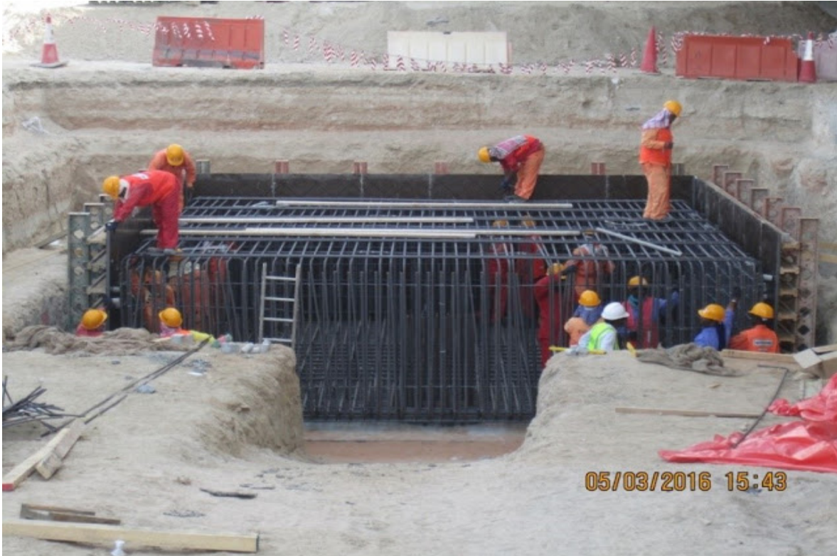
Fig.: 3.17. Reinforcement fixing for pile cap
