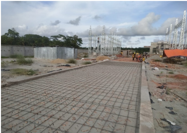
Fig: 4.8. Rigid pavement rebar placement
