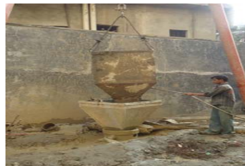
Fig: 3.8.Pouring concrete in the tremie pipe
