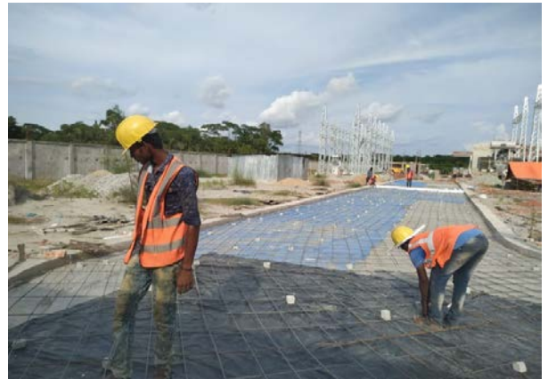
Fig: 4.9. Rigid pavement rebar placement
