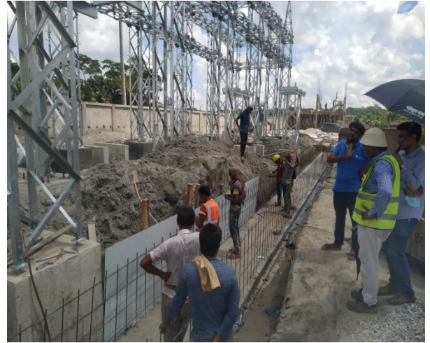
Fig: 4.13. Cable trench base & rebar binding
