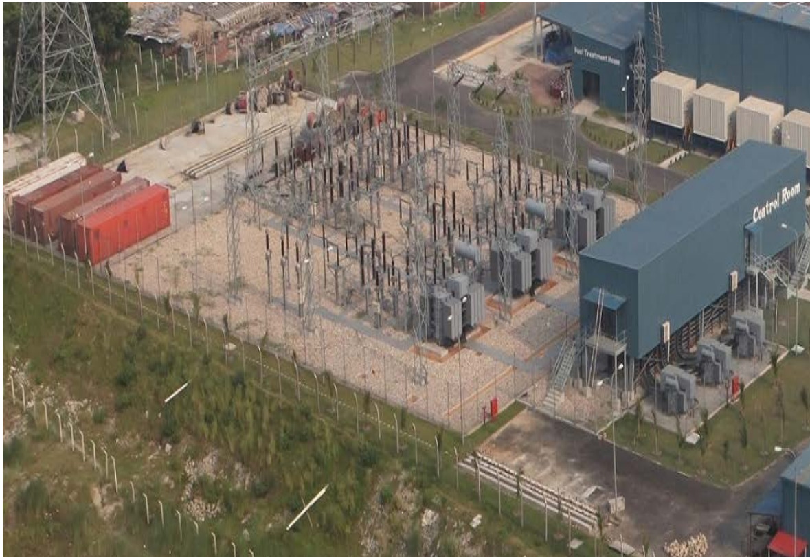
Fig.: 3.24. Landscaping and carry out the final inspection
