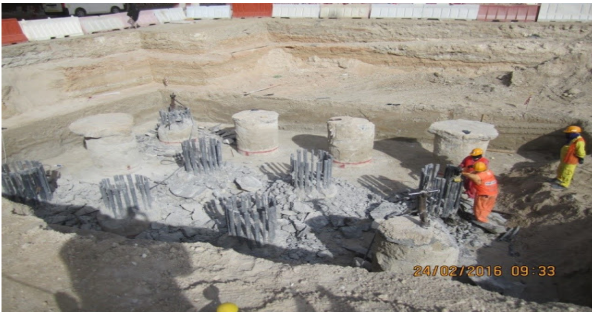
Fig.: 3.14. Pile head breaking
