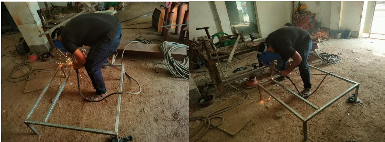
Fig. 7: Welding GI Square Frame.
