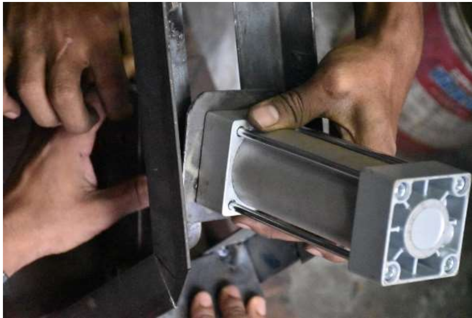
Figure 4.4: Installation of Pneumatic Cylinder
