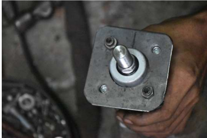
Figure 4.3: Installation of Pneumatic Cylinder
