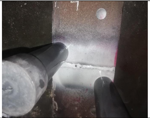
MPI of Welding Plate-4
