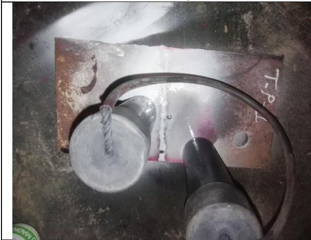
MPI of Welding Plate-1
