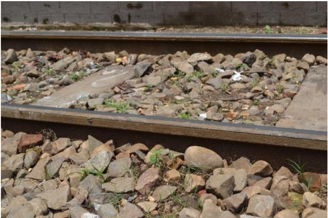
Figure 4- 4.28 Enough Stone under Line
