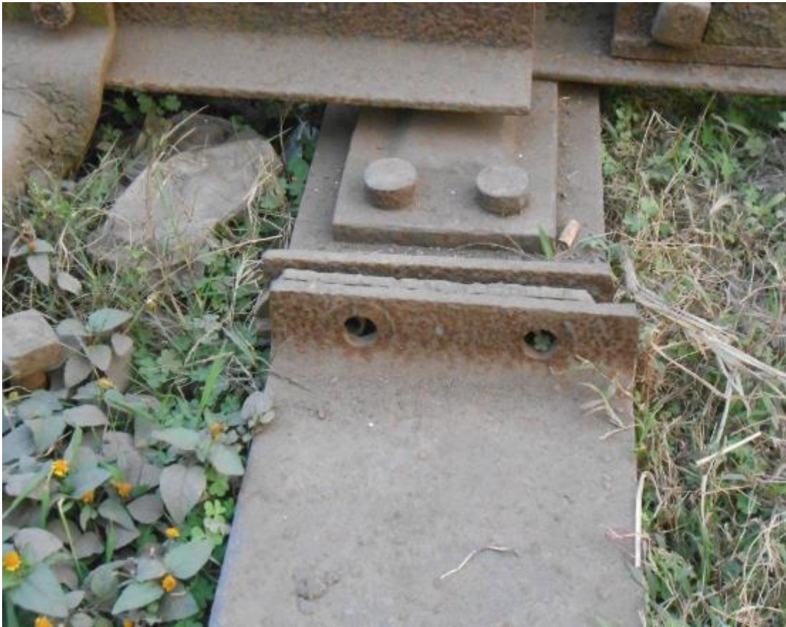
Figure 4- 4.62 Lacking of Bonding.
