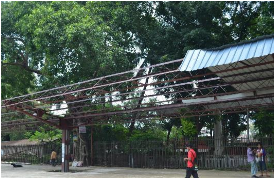
Figure 4- 4.24 Inadequate Protection for Passengers
