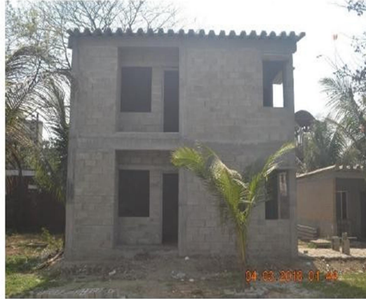
Figure 1.1.8 : Model House-II using Compressed Stabilized Earth Block and Thermal Block at HBRI campus
