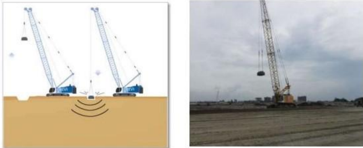
Figure 3.11: Execution of Dynamic compaction work. [7]
