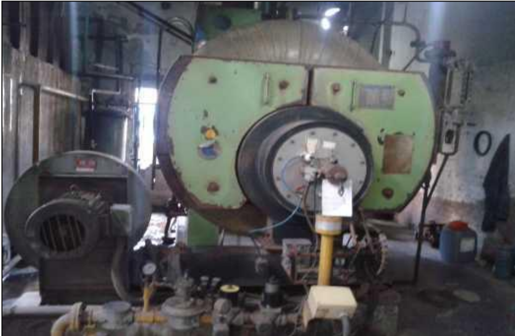
Fig: Cochran Boiler, Fire Tube
