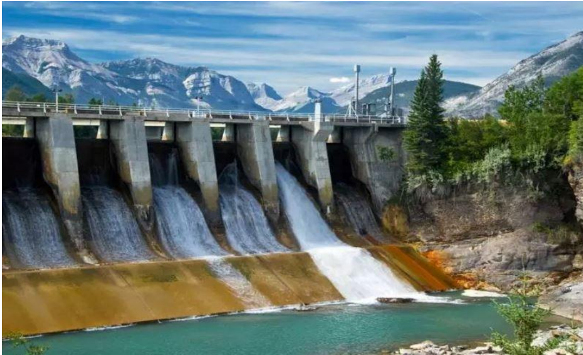
Figure 2.1 hydroelectric power plant.
