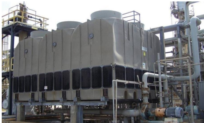
Figure 2.10-multi factory assembled cooling tower [10]
