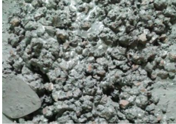
Figure 3.2: Preparation of Mixing of Cement and Aggregate
