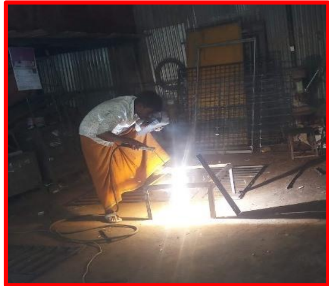
Figure 4.2 Welding Operation of MS Plate
