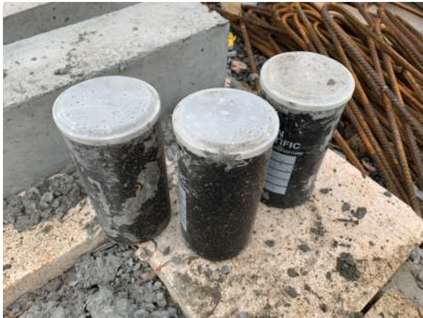
Fig 3.9: Casting concrete in cylinder.
