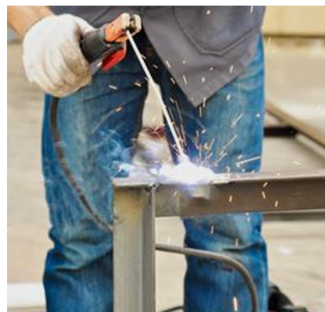
Fig: Welding operation
