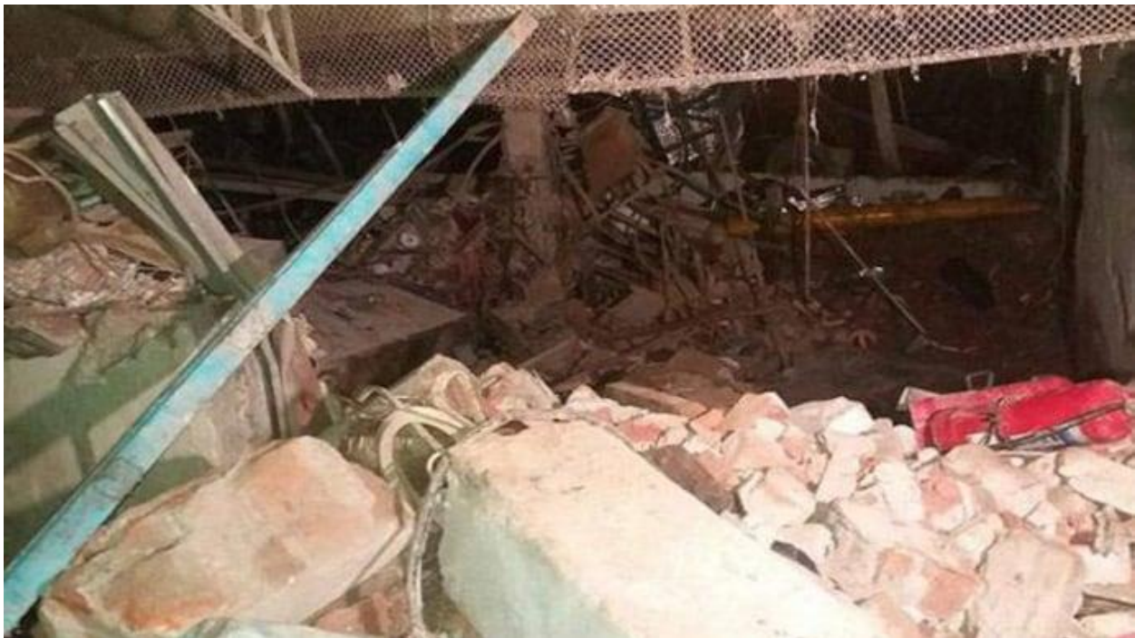
Fig.2.7: boiler explosion at a garment factory in Gazipur ( https://www.thedailystar.net/frontpage/boiler-blast-kills-four-gazipur-1427953 )
