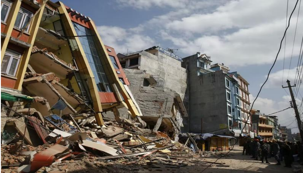
Figure 1.2: Earthquake damaged structures
