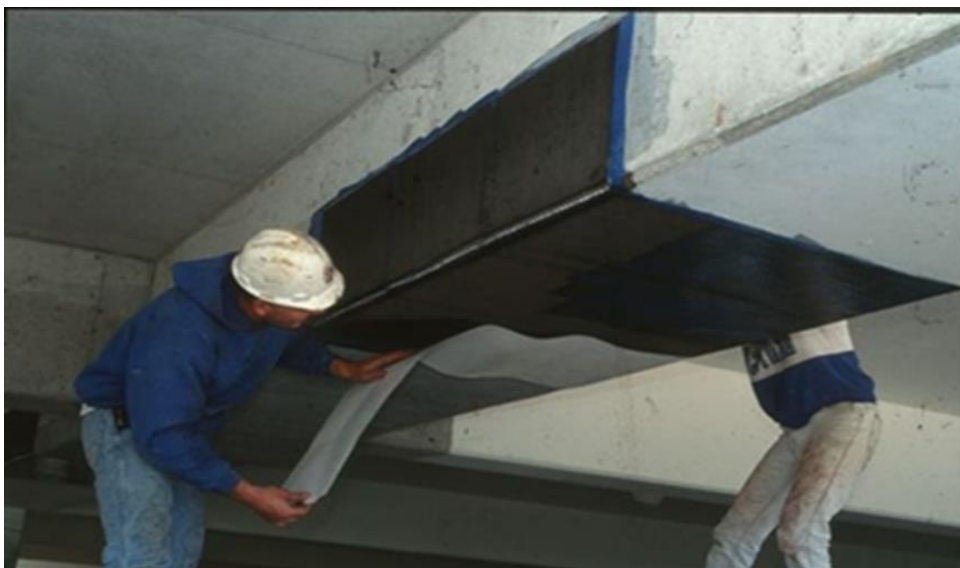
Figure 2.1: Strengthening process of RC beam using CFRP composites
