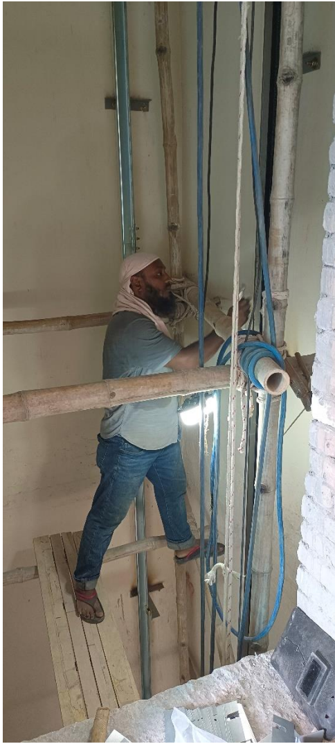
Figure 4-19. Workers working without lifting equipment (Shackles and Web Sling) and without helmet and no full body harness.
