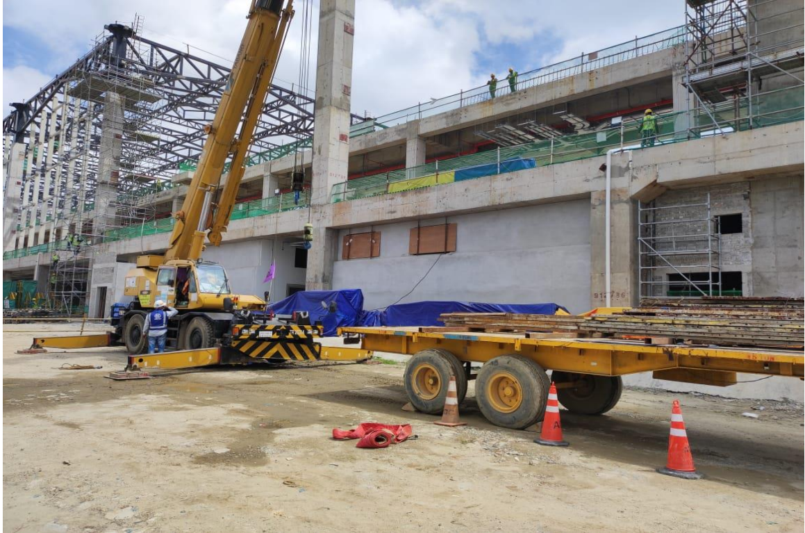
Figure 4-3. Arrangements of cranes in the Airport Terminal 3
