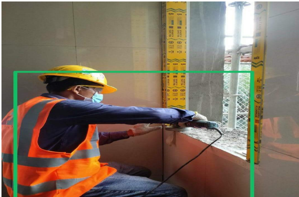
Figure 4-6. Grinding with proper safety (Line-6)
