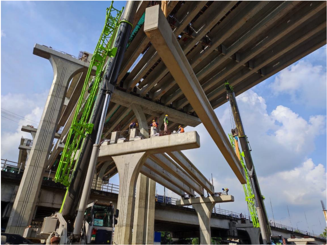
Figure 4-15. Proper safety should be implemented during heavy lifting
