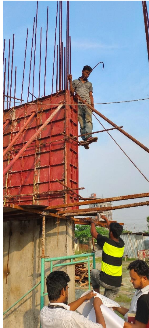
Figure 4-19. Workers working without lifting equipment (Shackles and Web Sling) and without helmet and no full body harness.
