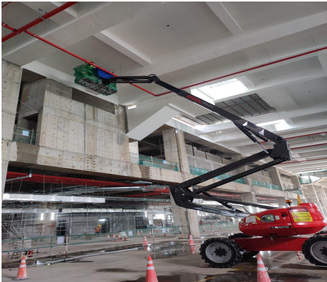
Figure 4-4. Bird Proofing, Netting installation (light lift) for Airport Terminal 3
