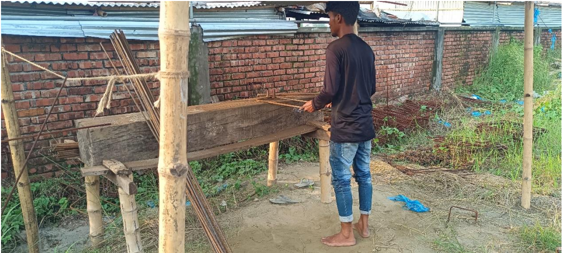
Figure 4-20. Worker engaged in rod cutting without safety helmet, gloves, boot and face shield.
