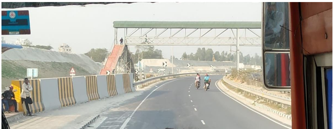
Bejgaon area over bridge
