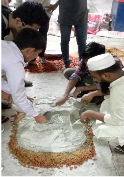
Figure 3.6: Concrete Mixing.
