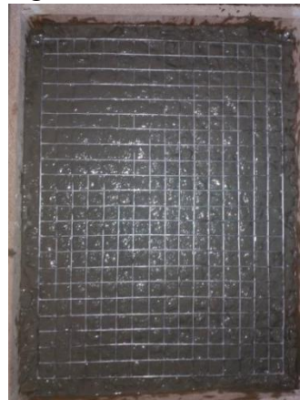
Figure: 2 nd Layer of Steel Wire Mesh Concrete Slab
