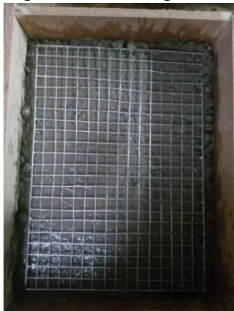
Figure: 1 st Layer of Steel Wire Mesh Concrete Slab
