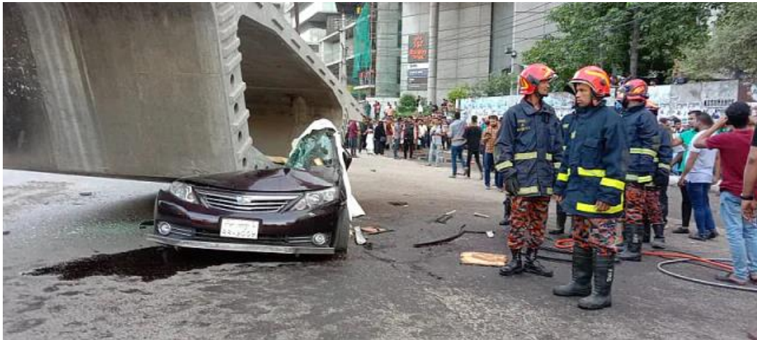
Fig 4.15: Accident due to authorities' fault (Initial Probe Finds Proof of Negligence in Dhaka BRT Girder Crash That Killed 5)
