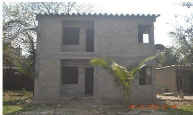
Figure 2.6 : Model House-II using Compressed Stabilized Earth Block and Thermal Block at HBRI campus
