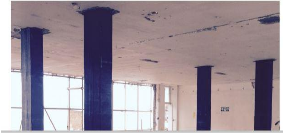
Figure 2:2 (1), (2), (3) Strengthening process of RC column using CFRP composites
