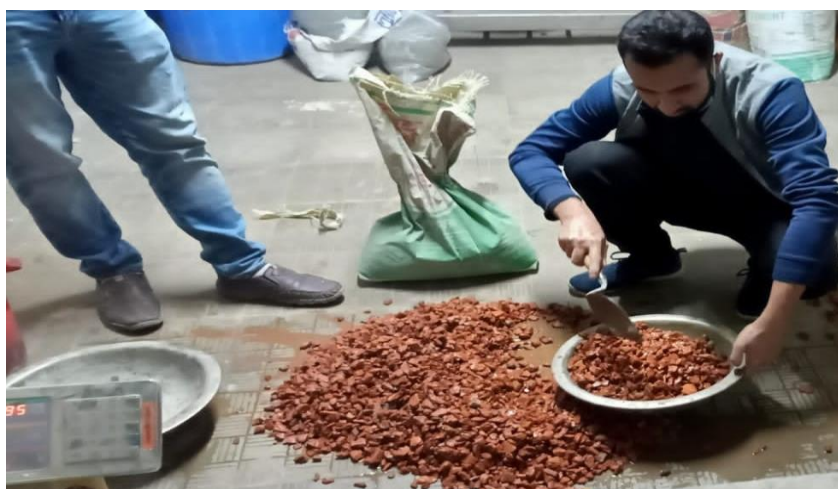
Fig. 3.2: Mixing of Sand Cement and brick chips.
