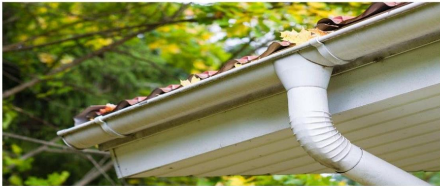
Figure 2-7: Gutters and Down take pipe [7]
