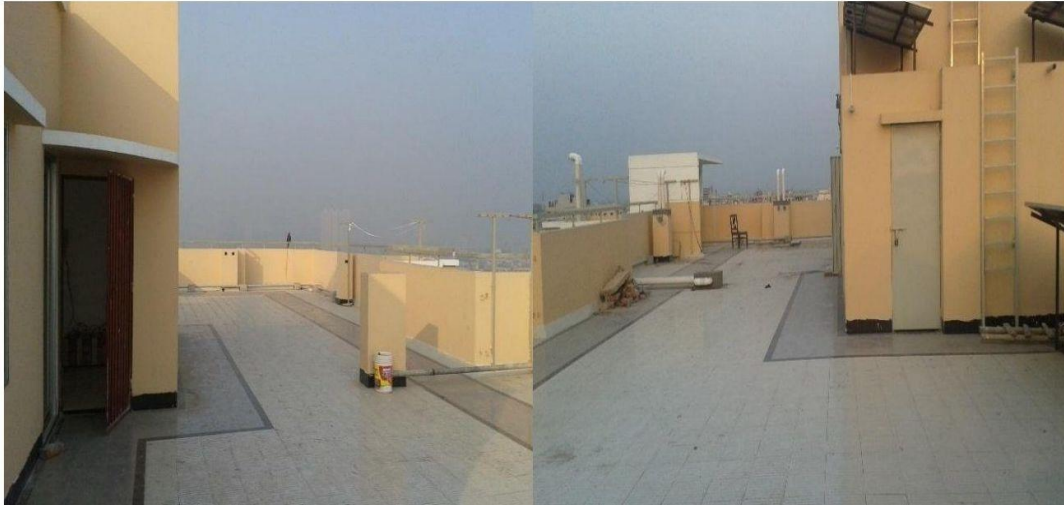
Figure 3-10: Rooftop of study project building at Dhanmondi
