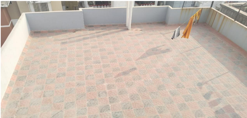
Figure 3-4: Roof top catchment area of this project
