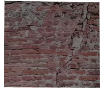
Fig 10: Damaged Bricks
