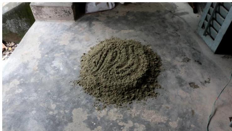
Fig 4.43: Lime Sand Plaster Preparation
