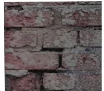
Fig12: Efflorescence
