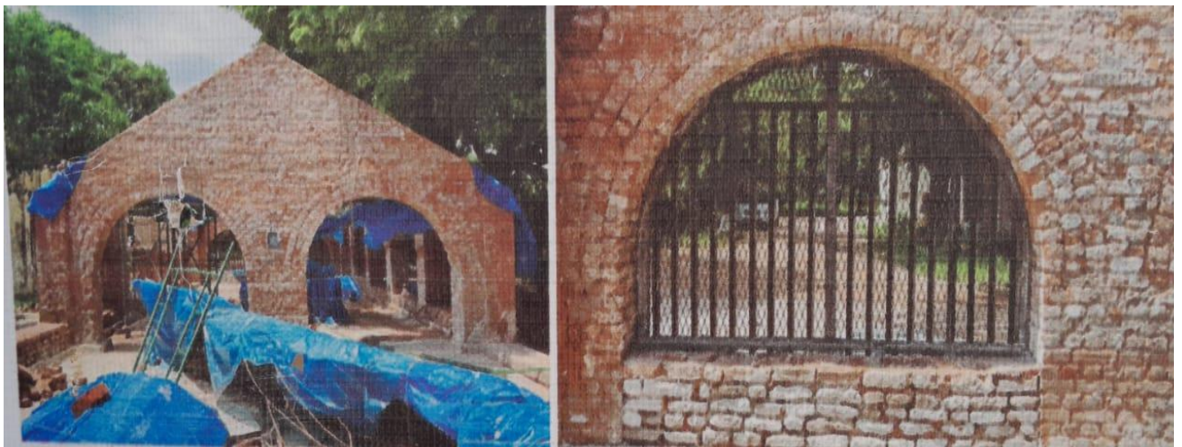
Fig 4.29: De-Plastering
