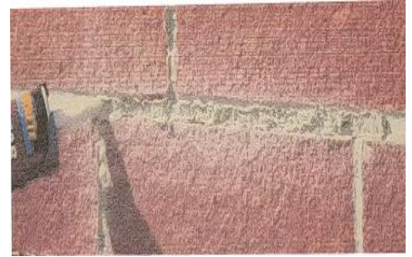
Fig 20: Patching in brick wall
