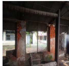
Replacing broken Brick with same size brick
