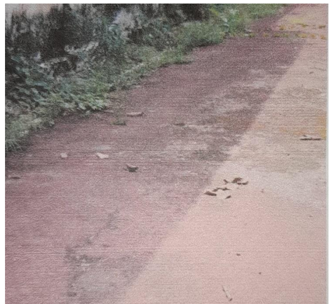
Fig 4.2: Pavement Beside Workshop 01
