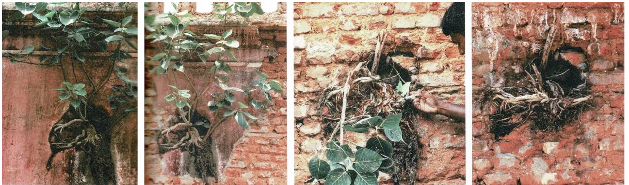
Fig 4.24: Strangler Fig Plants or Trees in Building
