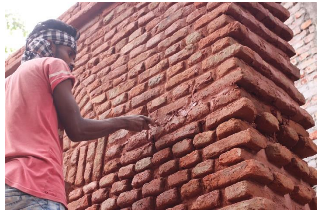
Fig 4.40: Process of Recessed Pointing (Maintaining the Old Brick Wall)
