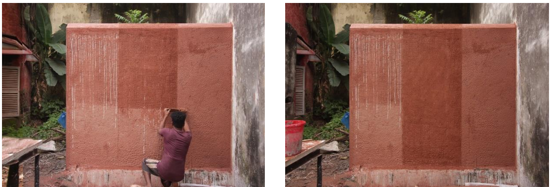
Fig 4.42: Lime Surki Plaster Process
