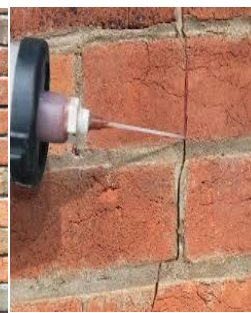
Fig 4.33: Repairing the Cracks
