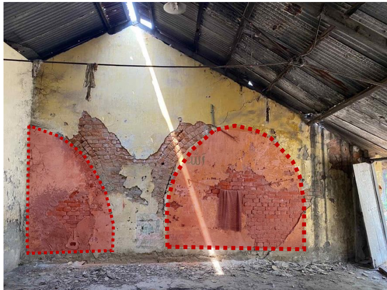
Fig 4.28: Arched opening revitalization from CP05
