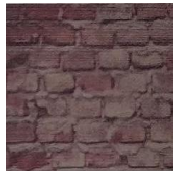
Fig 11: Unsuitable Pointing
