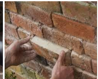
Replacing broken Brick with same size brick
