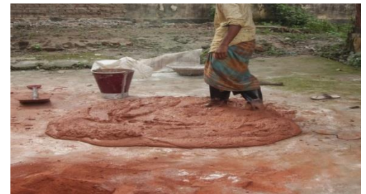
Fig 4.36: Preparation of Lime Surki Mortar
