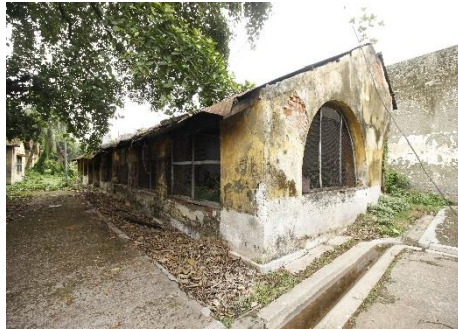
Fig 4.25: Existing Wall Condition
