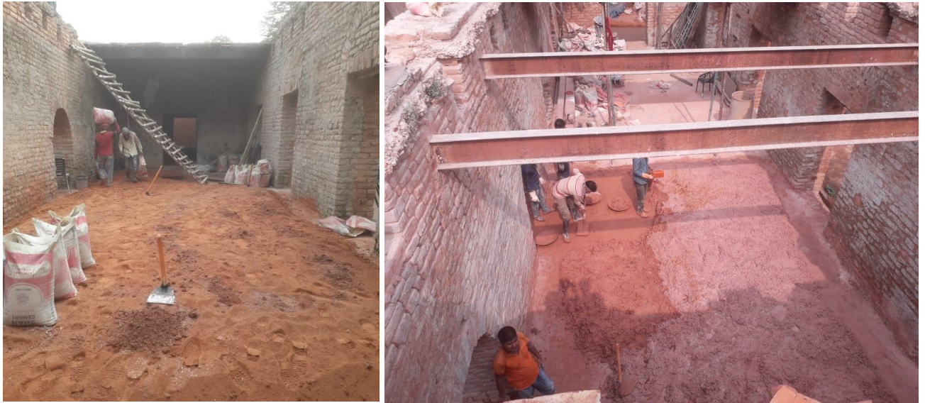
Fig 4.46: Lime Concrete Mixing
