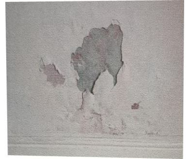
Fig 14: Damped Plaster
