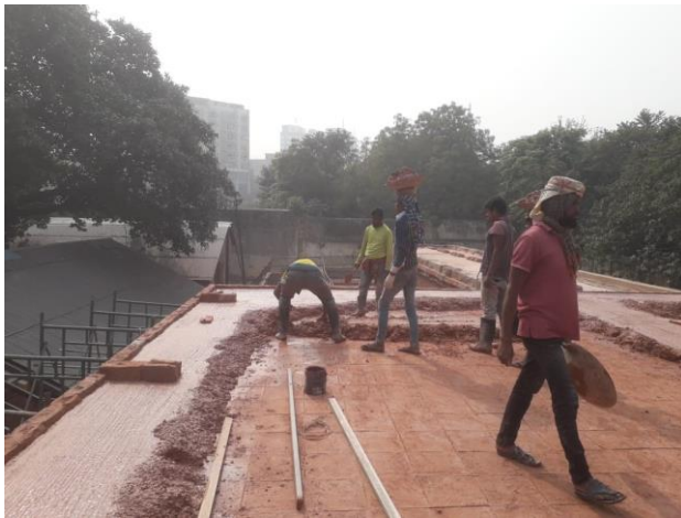
Fig 4.47: Lime Terracing
