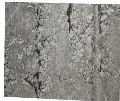
Fig 16: Honeycombed Concrete
