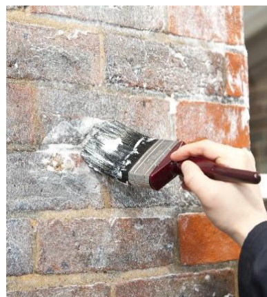
Fig 4.32: Damp Proofing Works
