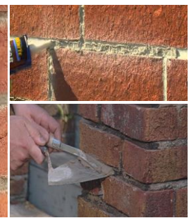
Replacing broken Brick with same size brick
