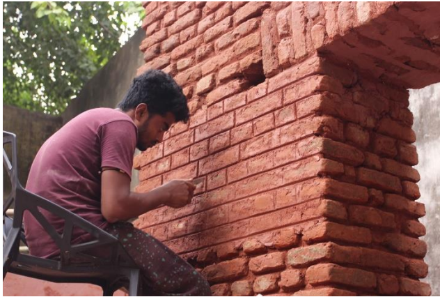
Fig 4.39: Process of Rope Pointing
