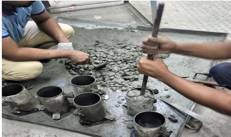
Figure 3.5: Compaction of the concrete
