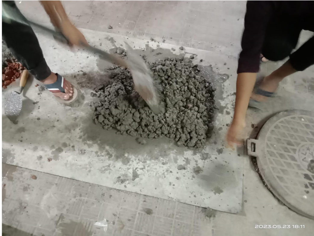
Figure: 1.14 Concrete Mixing
