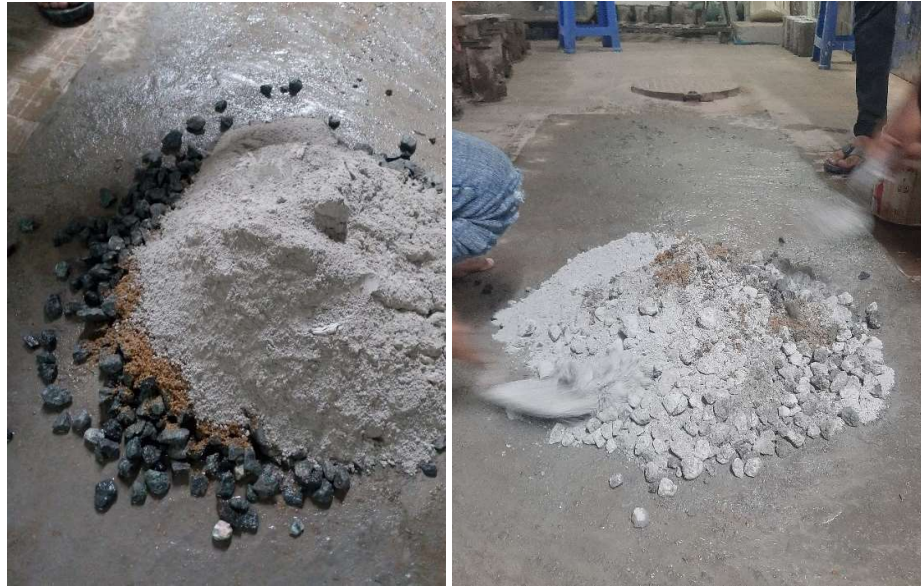
Fig 3.5: Ordinary (Control Mix) Concrete Mixing with Traditional Materials
