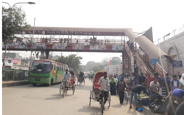
Figure 4: Hawkers in front of foot over bridge 1
