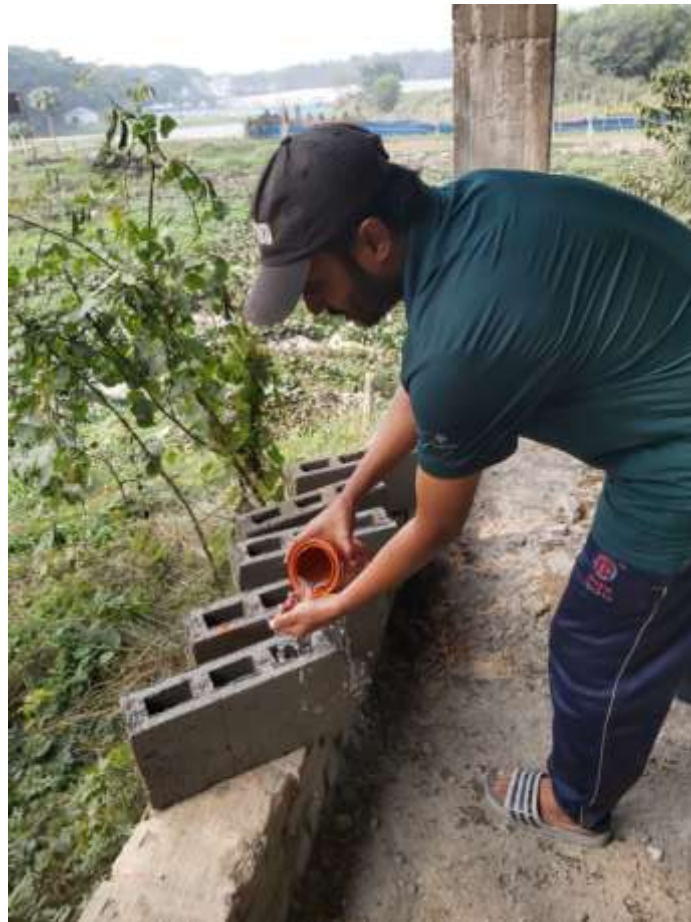
Figure: 1.9 Block Curing
