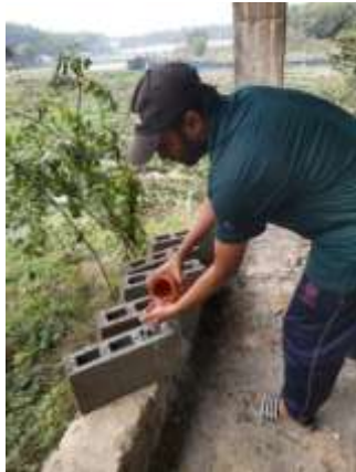
Figure: 1.9 Block Curing
