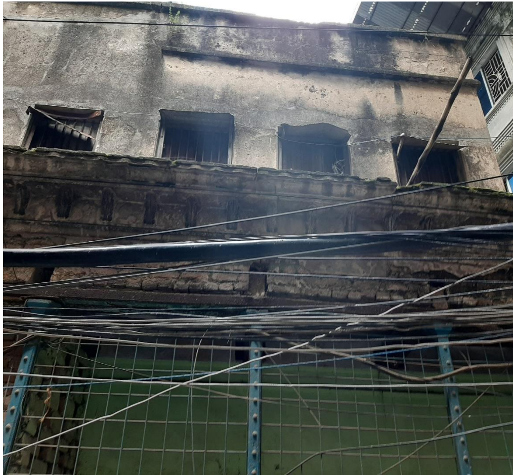
Figure.4.17. Front side view of the building.
