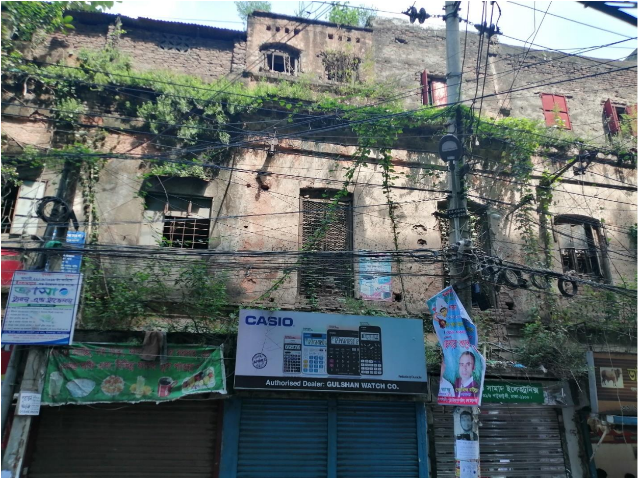
Figure.4.11. Front view of the building.
