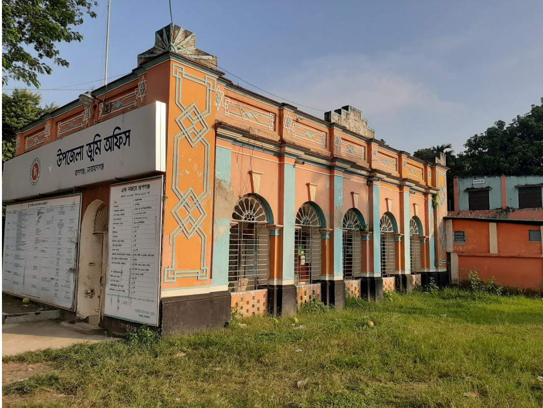
Figure.4.9. Front view of the building.
