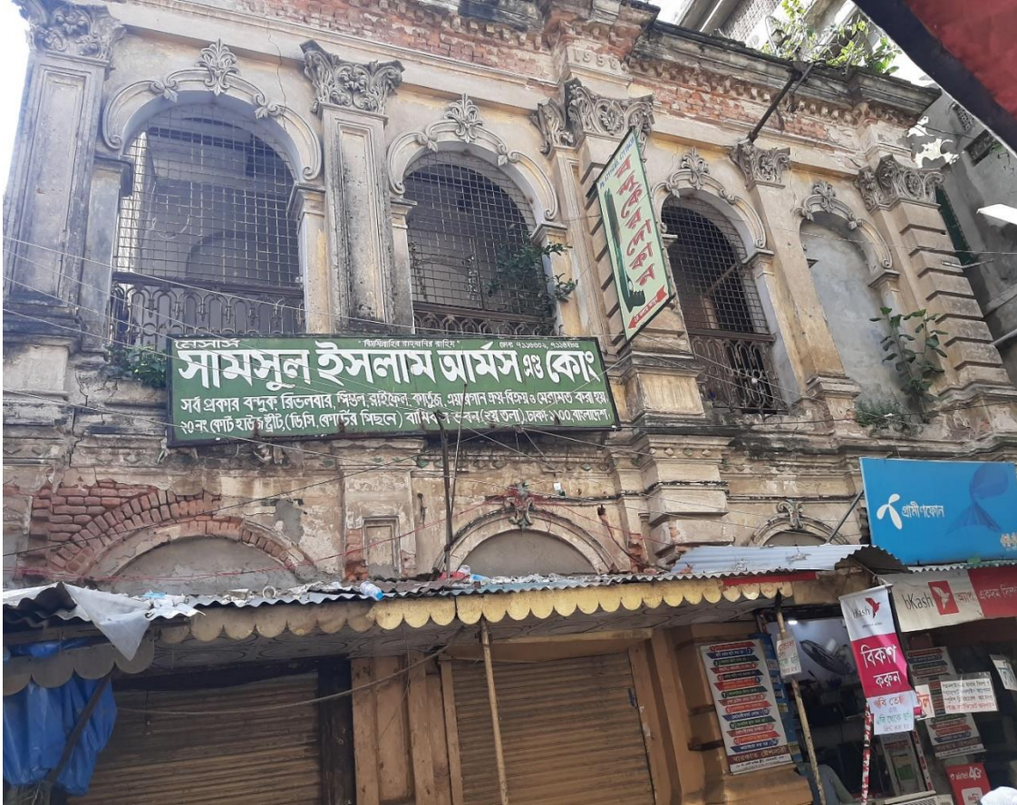
Figure.4.19. Front side view of the building.
