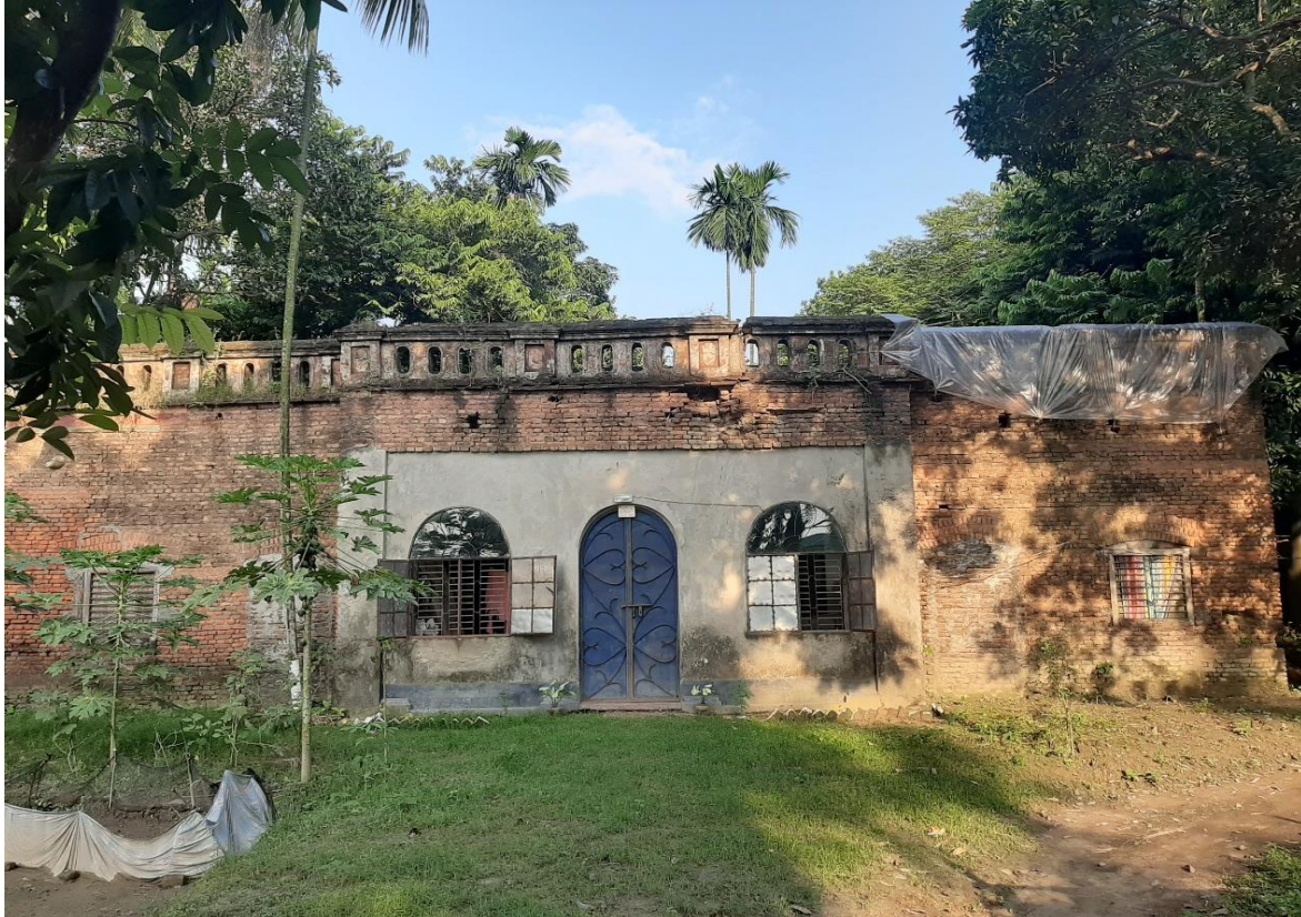
Figure.4.7. Front view of the building.
