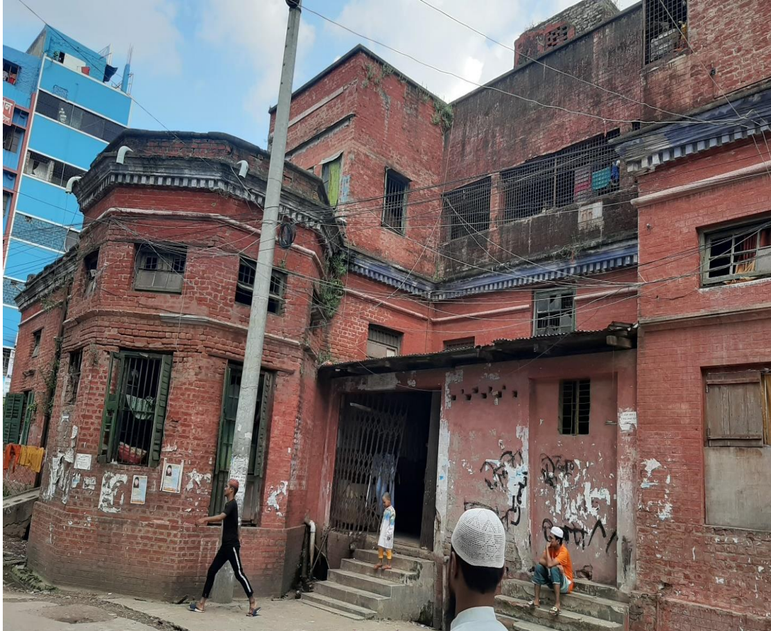
Figure.4.13. Front view of the building.
