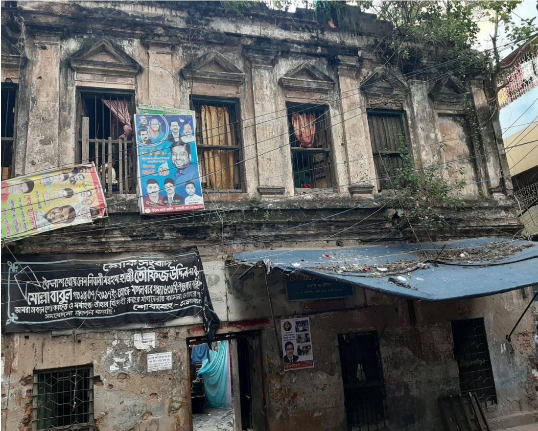
Figure.4.15. Front view of the building.
