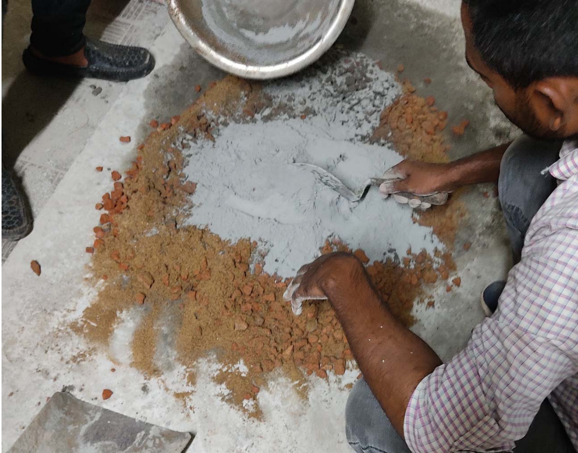
Figure 3-2. Mixing of Sand, Cement & Brick Chips
