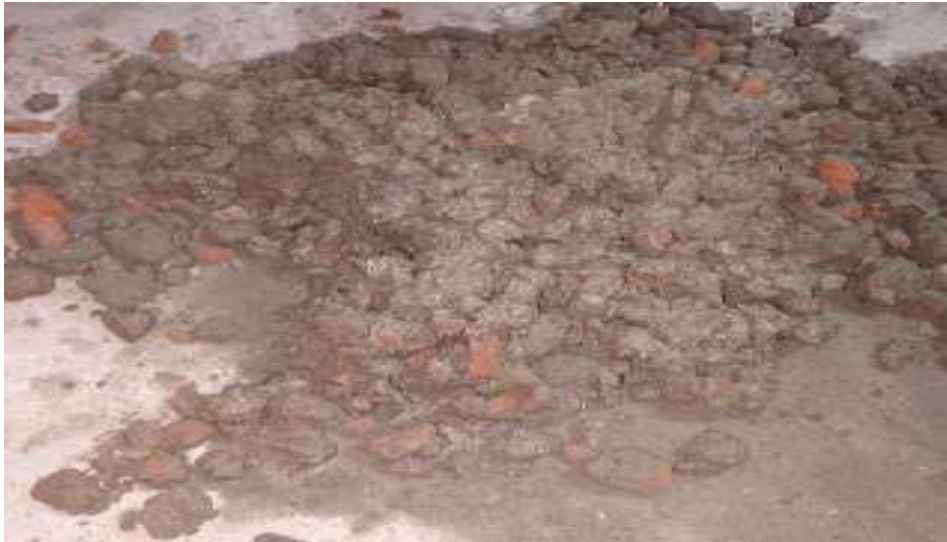
Figure. 3.9 mixing of concrete
