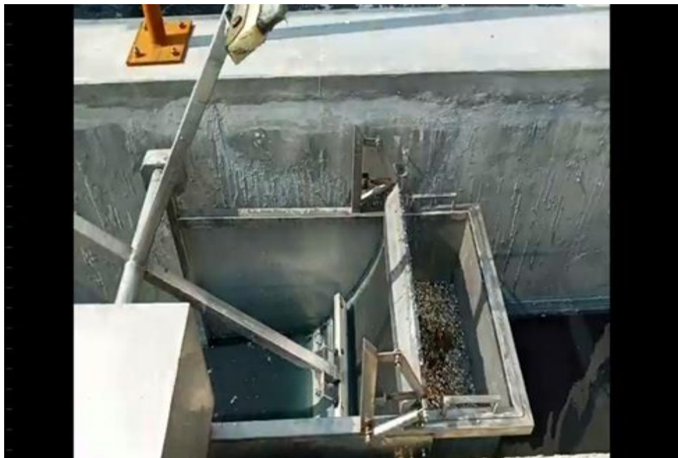
Figure 3.5: Sludge thickener
