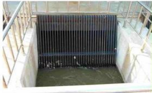
Figure 2.4: Screen Chamber
