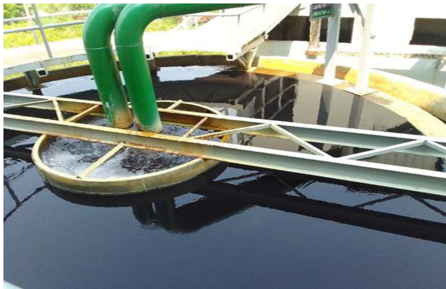
Figure 3.3: Clarifier Tank 2
