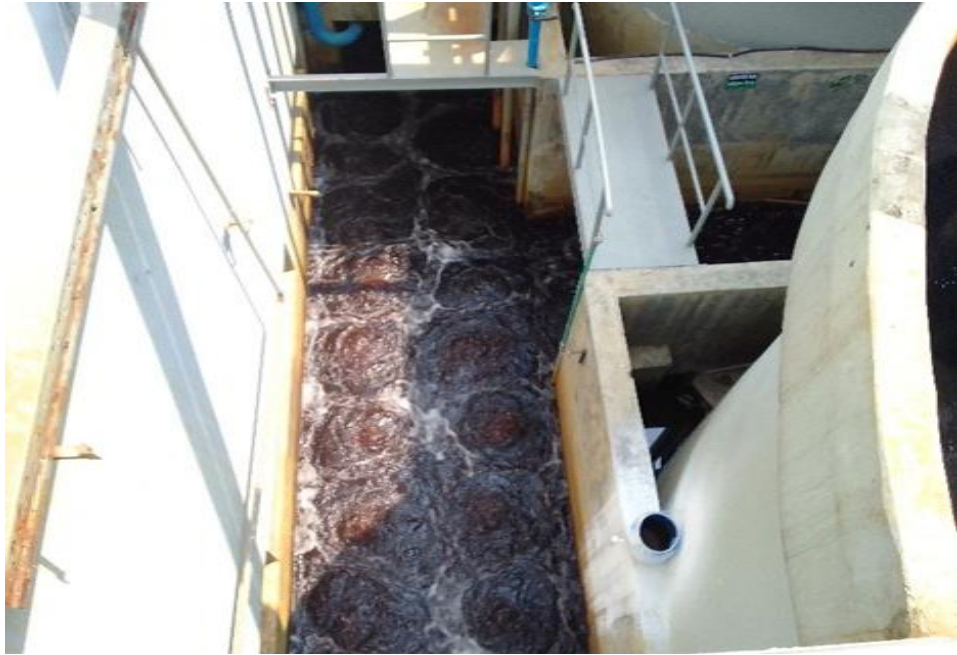
Figure 3.4: Equalization tank
