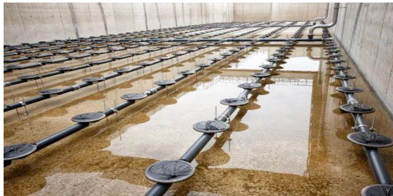
Figure 2.8: Diffuse Aeration
