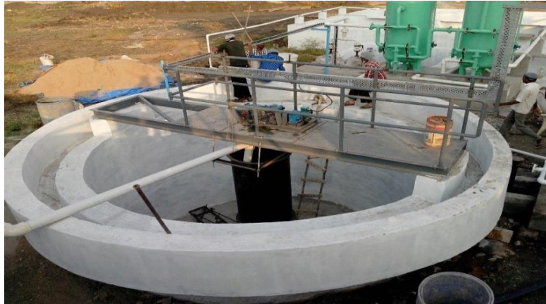
Figure 2.9: Secondary Clarifier
