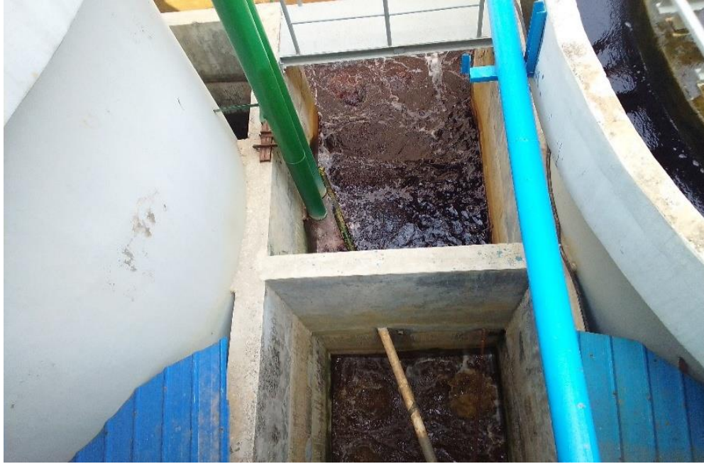
Figure 3.6: Oxidation tank
