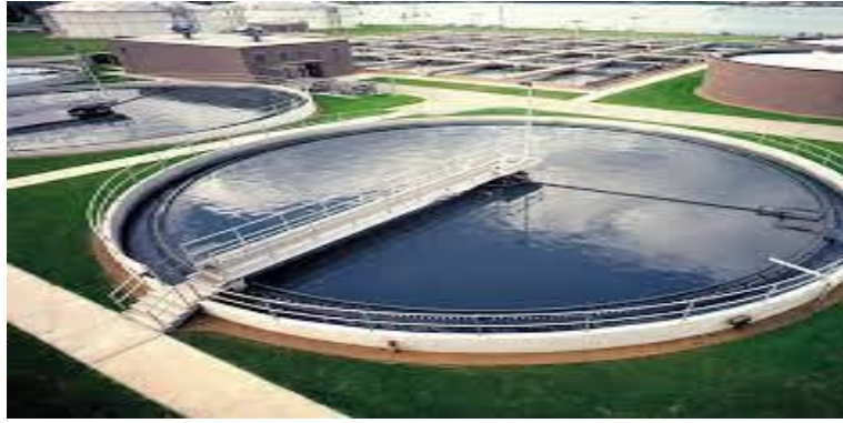
Figure 2.7: Primary Clarifier
