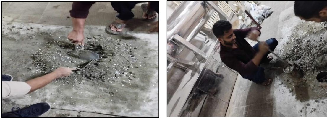
Fig. 3.11: Concrete mixing & pouring
