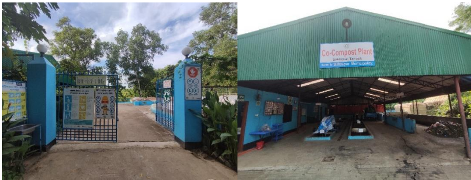
Figure 1- 2. Sakhipur Fecal Sludge Treatment Plant
