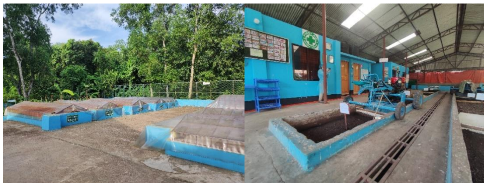
Figure 2- 6. Co-composting Plant in Sakhipur, Bangladesh
