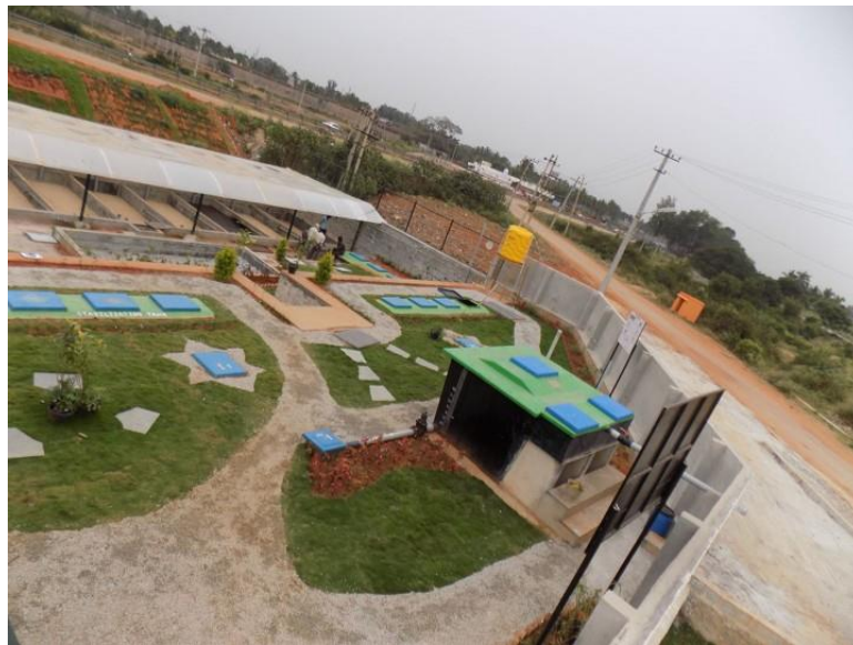
Figure 2- 5. Devanahalli Fecal Sludge Treatment Plant (FSTP), India
