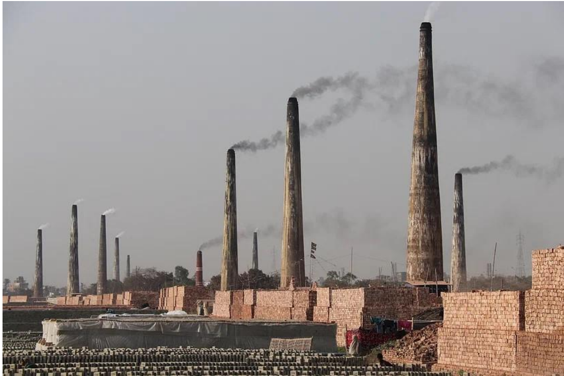
Figure 3-1: Chulli of Traditional Burnt Clay Bricks
