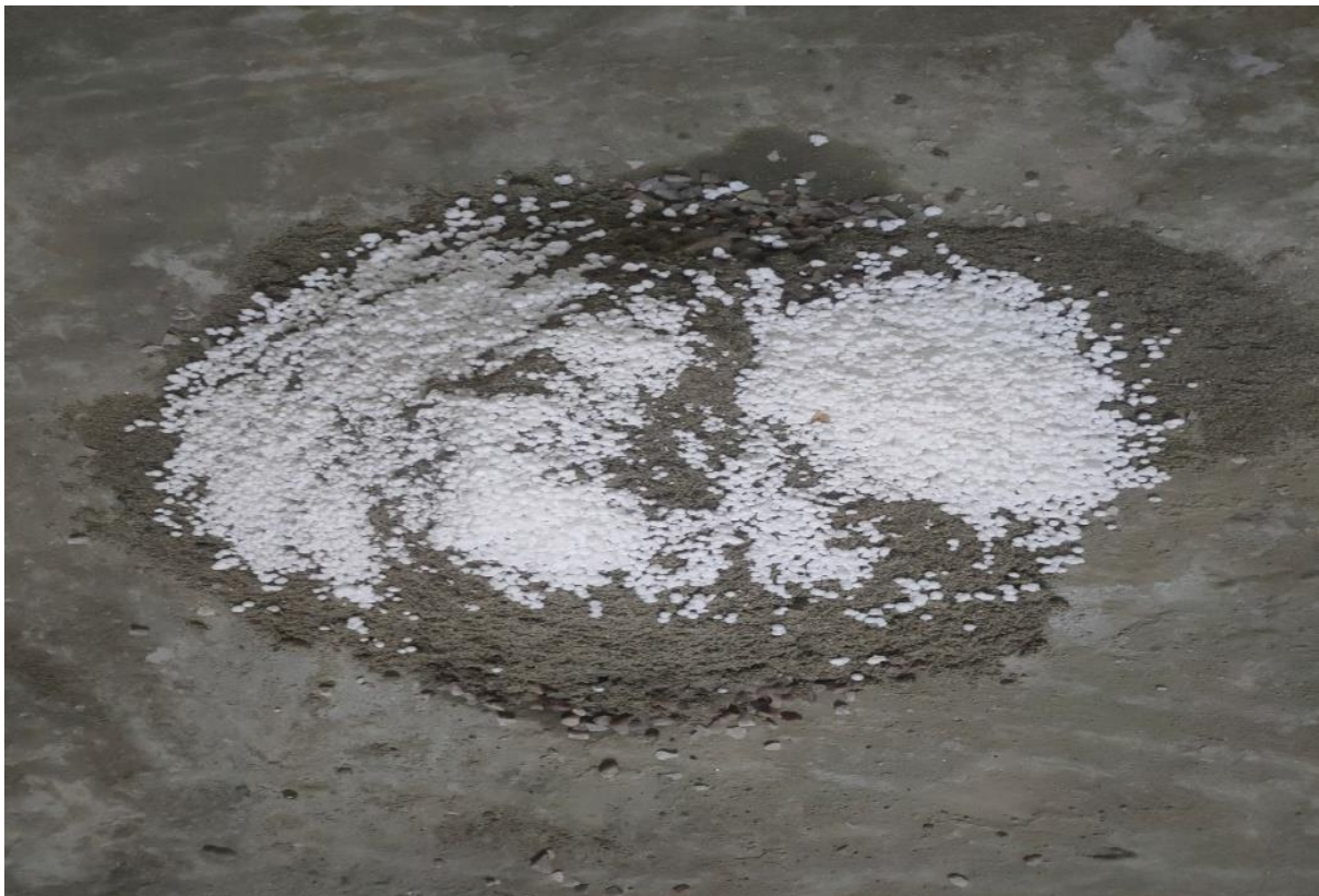
Fig: 3.4.1 Mortar mixing.
