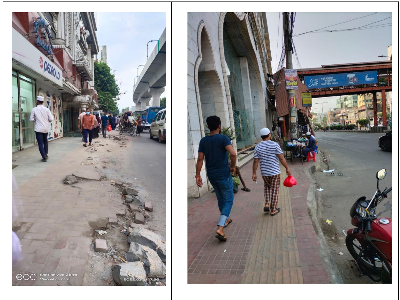
Figure 3-12. During footpath condition survey
