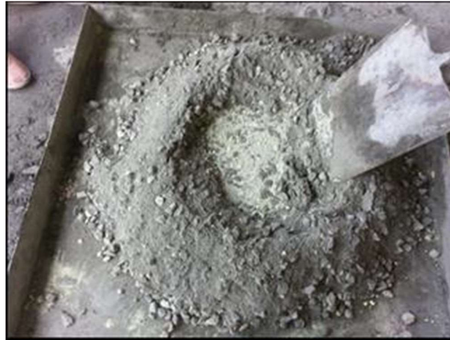
Figure 3.3 Manual mixing
