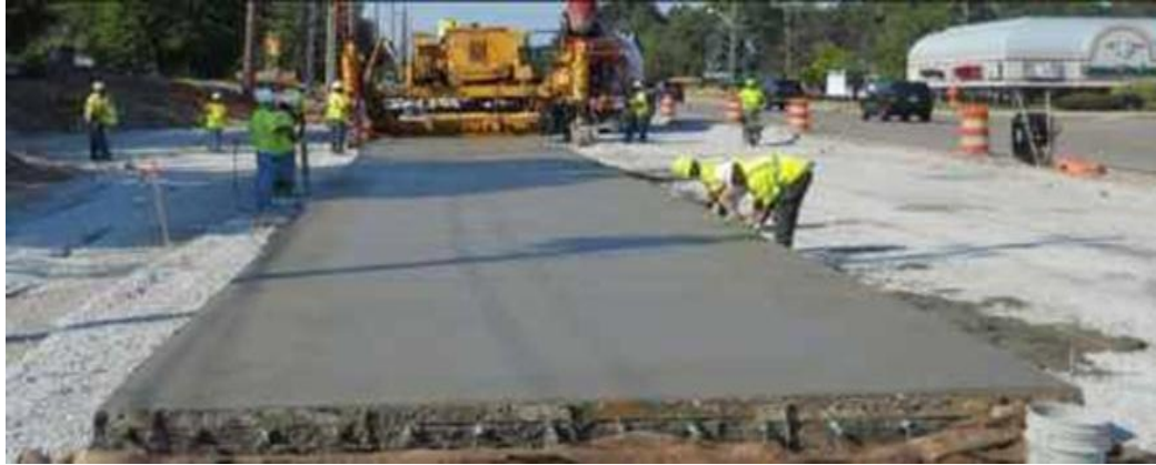
Fig 2.2: Concrete Slab Laying [14]
