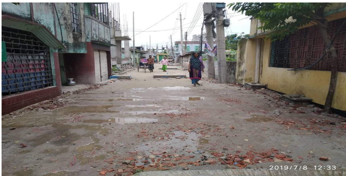
Fig 2.3: Providing Base Course (WBM)
