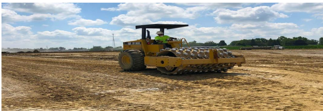
Fig2.5: Soil compaction of road construction [16]
