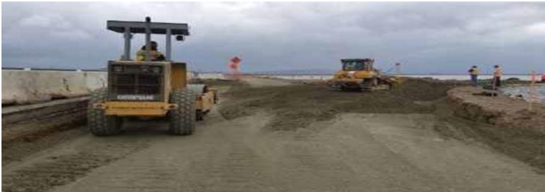
Fig 2.4: Laying of Sub base Course [15]
