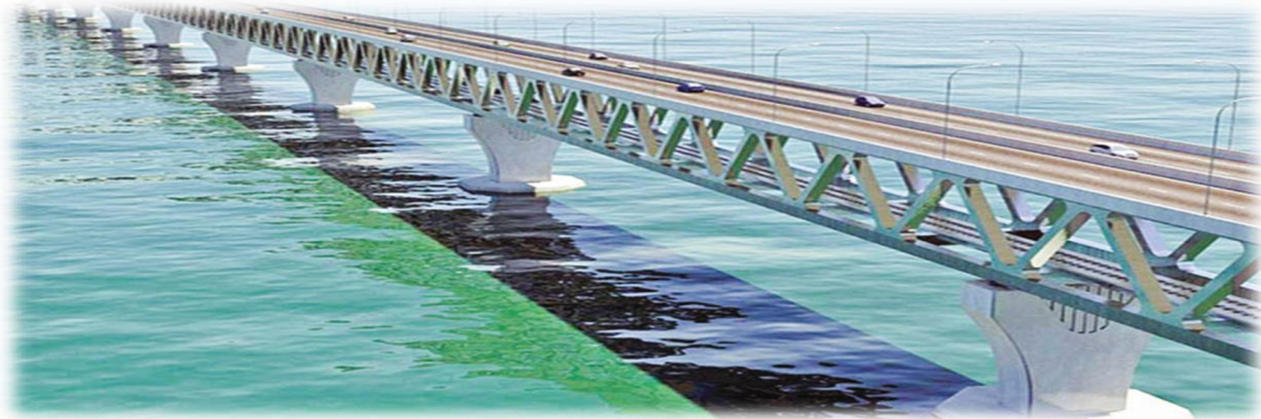
Figure: Padma Bridge
